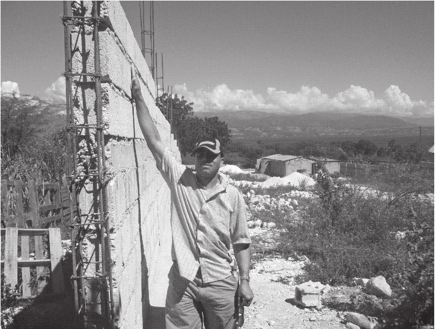
Jean Volcy, an elder of the Strathmore Boulevard Church of Christ, stands beside a portion of the security fence that is part of the work under construction in Fond-Parisien, Haiti. See his report on the progress this Haiti Mission on page 14.
